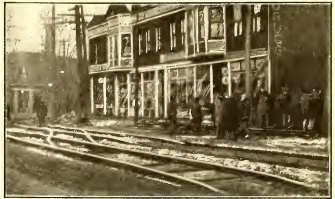
VIEW OF PORTION OF TEMPORARY TRACK WORK
